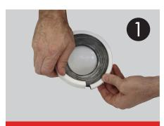
Cut and remove leaking pan collar rubber.
