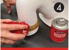
Clean off excess wax with Silicone CleanUp or suitable solvent.
