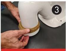
Cut and insert wax seal into pan collar, push in and smooth to shape.
